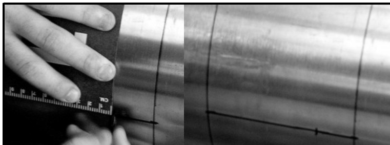
Figure 28: Measuring and Marking Spacing
