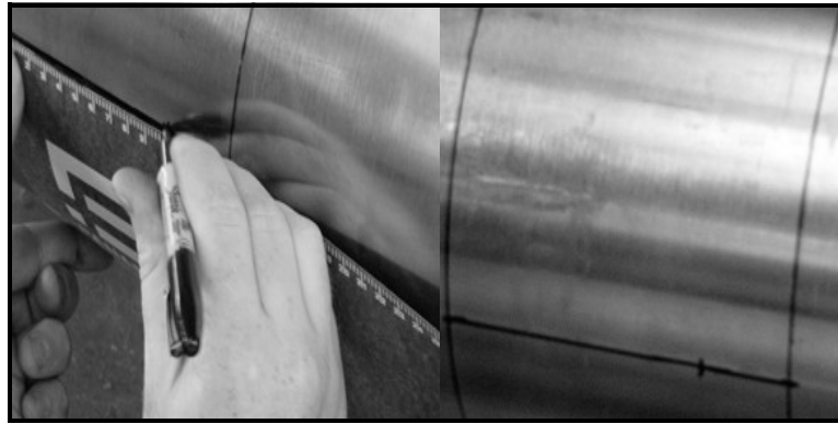
Figure 24: Marking the 9 o'Clock Position
