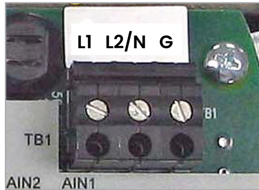
Figure 20: Wiring the AC line power
