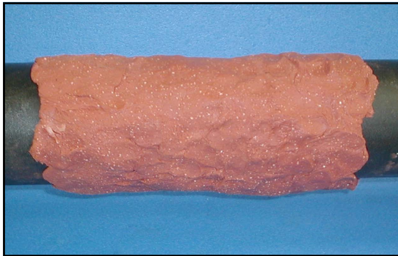
Figure 9: Spreading DMP-3 Damping Material
