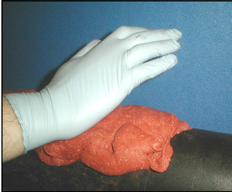
Figure 8: Applying DMP-3 Damping Material
