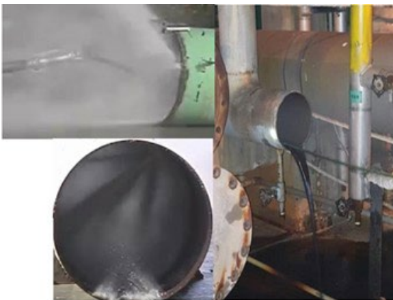
Figure 8. Water washing and purging on the pipe
