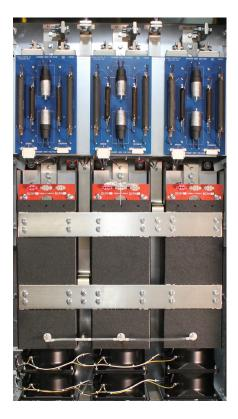
Systems include AC input fuses, snubber circuits, conduction sensing, new gate firing interfaces, and power cable terminations. Power auxiliaries like input/output breakers or contactors can be replaced as extended scope options. Where an added level of reliability is required, the new power converters can be supplied with redundant cooling fans or simplex systems may be upgraded to fully redundant power converters where space allows.
