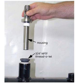
Figure 12: Inserting housing into pipeline
